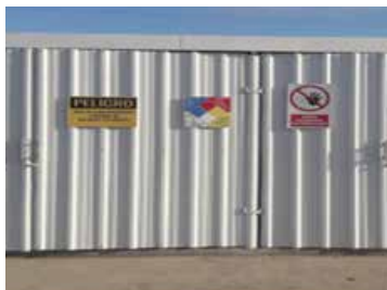
► HAZARDOUS WASTE A new space for Hazardous waste was built, allowing an adequate segregation of waste , containment of possible spills and compliance with safety measures.
